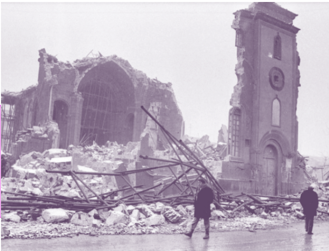
Sputnik. The Church of Christ the Saviour in Leninakan after the earthquake in Armenia on 7 December 1988.
